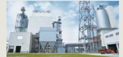
Mombetsu Biomass Power Plant
