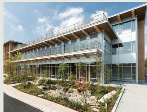
New research building at Tsukuba Research Institute
